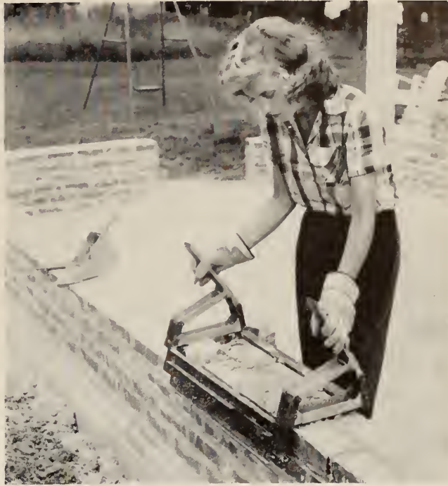
New bricklaying device saves many man-hours. —Wide World Photo.
